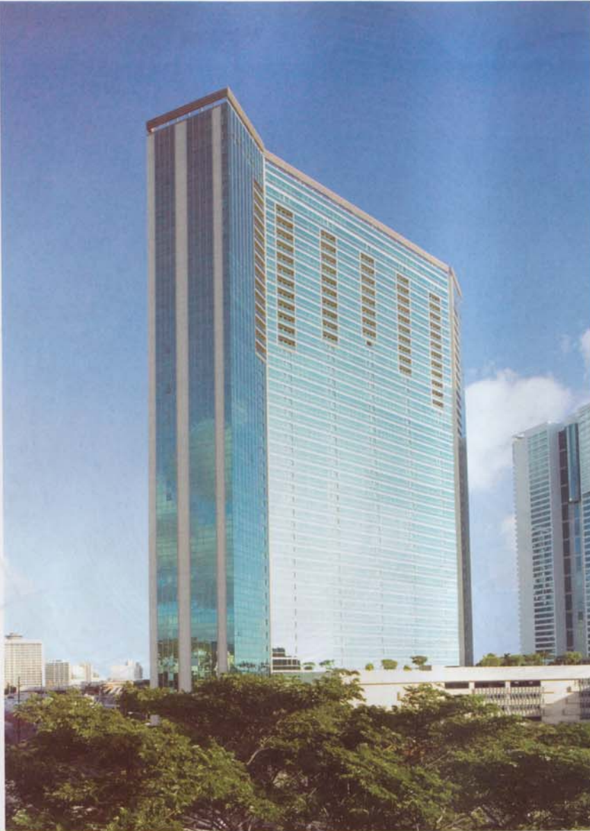
THE 48-FLOOR KO'OLANI IN DOWNTOWN HONOLULU USES INSULATED GLASS. SOUNDPROOF DRYWALL AND ACOUSTIBLOK LINING TO ACHIEVE STATE-OF-THE-ART NOISE REDUCTION FOR THE 370 STATE-OF-THE-ART LUXURY CONDOMINIUM.
